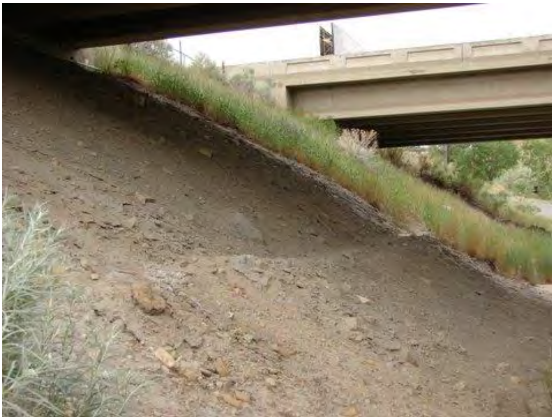
Figure 5. Highway bridge over a county road on US 6 near Price, Utah. This bridge will be provided with fencing to funnel wildlife under the highway. The path was created by wildlife crossing under the structure. Photo by Ruediger.
