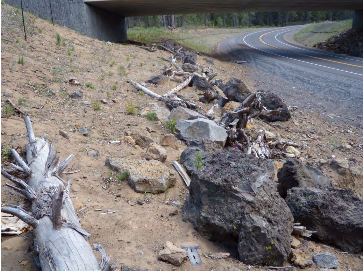
Figure 7. The Lava Butte project south of Bend, Oregon incorporated a wildlife lane into an existing underpass that was originally for vehicle use only. Logs and boulders were added to promote wildlife use. Photo by Jacobson.
