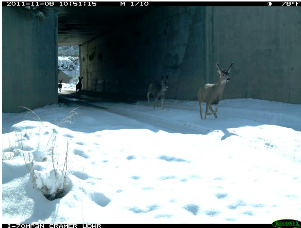
Figure 6. Deer crossing under I-70 in Utah. A number of Forest Service roads crossed the highway and have been fenced so deer can safely cross. Deer and elk collisions have been reduced from several hundred a year to almost zero. Photo by P. Cramer and UDOT.
