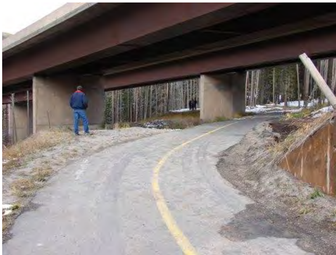
Figure 9. Bike path and trail going under I-70 near Vail Pass in Colorado. The multi-span bridge provides plenty of space for bikers, hikers and wildlife to pass under the highway. Photo by Ruediger.
