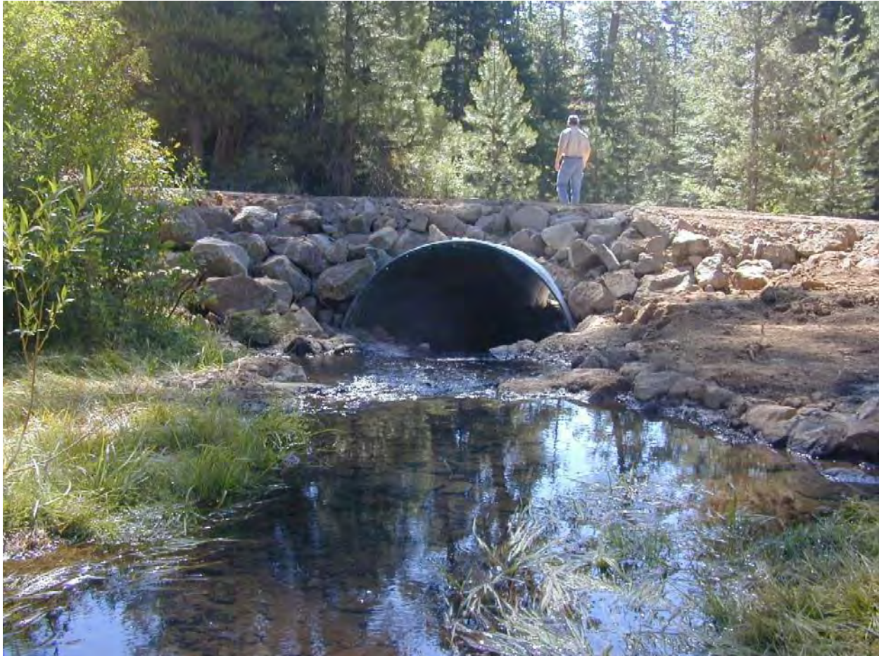
Figure 4. Good example of a "culvert replacement" arch on the Fremont-Winema National Forest. This structure greatly improves aquatic organism and small mammal passage. US Forest Service photo.
