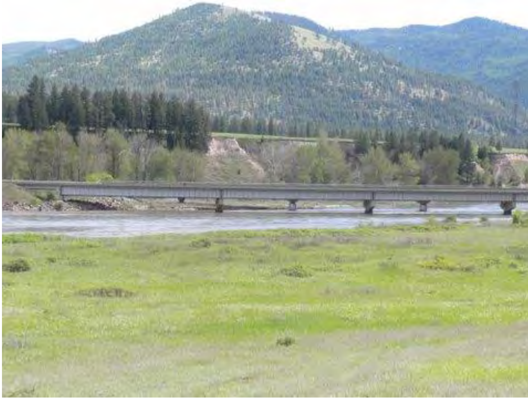
Figure 1. One of two span bridges on I-90 near Nine Mile exit that provided habitat connectivity for many species including wolves and grizzly bears. This fencing was modified by Montana Department of Transportation to facilitate wildlife movement. Photo by Ruediger.
