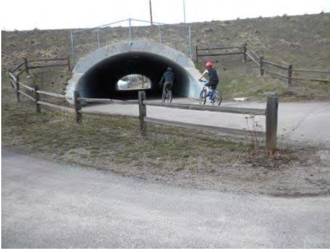
Figure 8. A trail and bike path bridge under a 4-lane highway in Missoula, MT. Is adequate in size to provide for deer, black bear and other smaller mammals. Photo by Ruediger.
