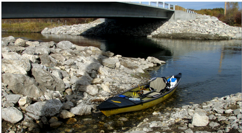
Bridge Access, East Gallatin River, Mike Cline
