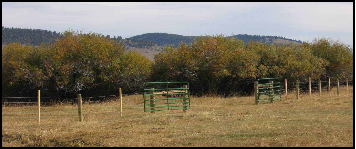
Openings, crossings, and passes incorporated into your fencing system allows for easy wildlife passage. In some situations or seasons, providing temporary passage across a section of fence may be the best solution to allow seasonal wildlife passage, as can be seen in this picture from a pasture along the Big Hole
